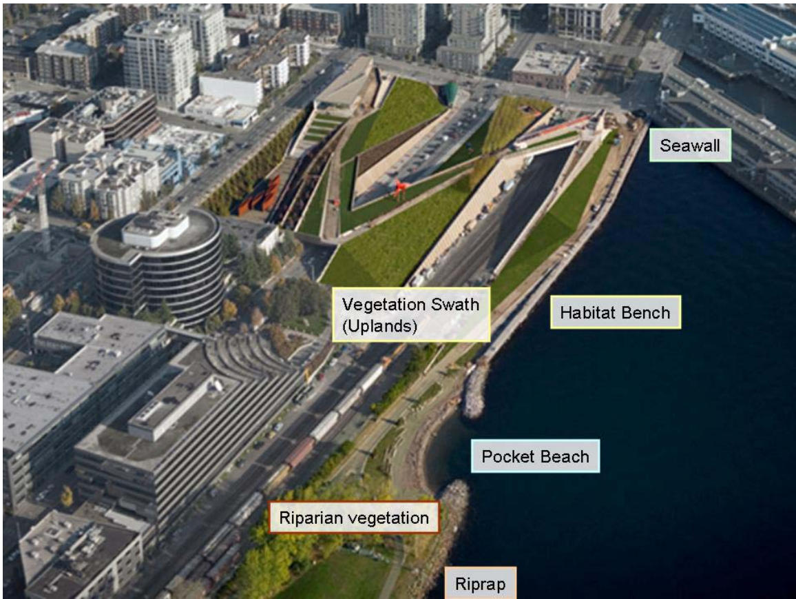
Aerial view of the Olympic Sculpture Park site after construction, showing general sampling locations.
